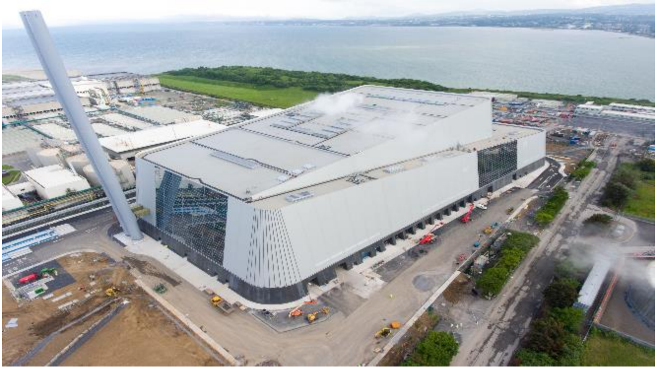
Site Aerial View Looking South East May 2017 (Copyright PML).
